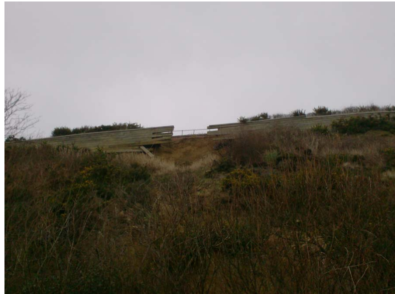
The collapsed cliff top and failed old timber revetment
