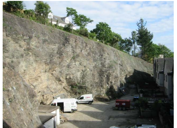
Rock netting tightly contoured with tensioned cable cross strapping
