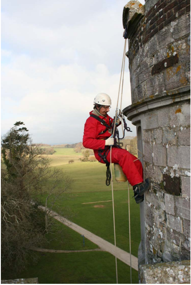
Vegetation removal and weeding
