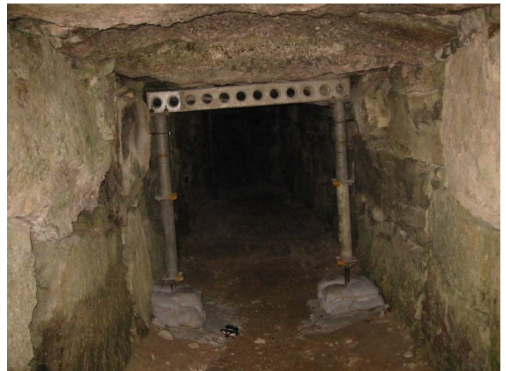
Access tunnels were assessed and where necessary, reinforced with props.
