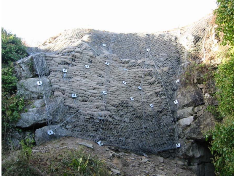
Stabilised dry stone retaining wall
