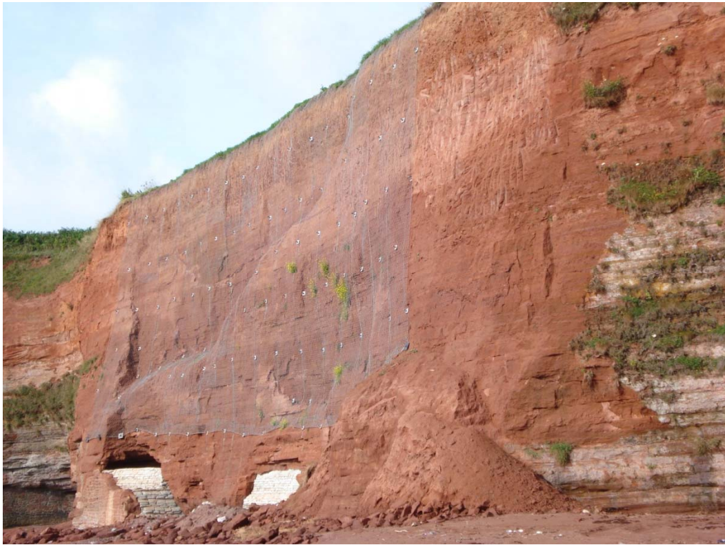
The rock face scaled, netted and bunds part built
