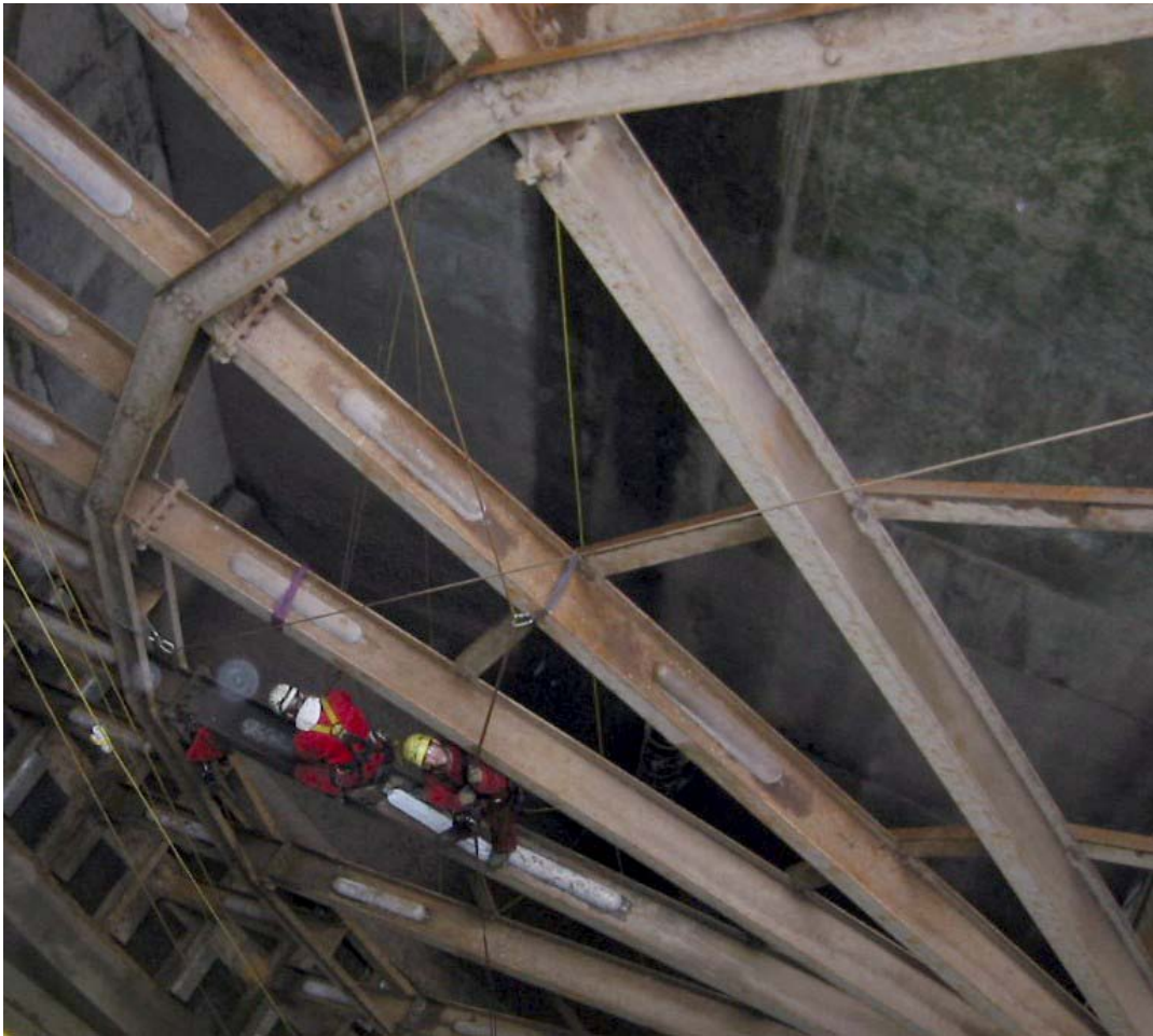
Installation of anodes.
