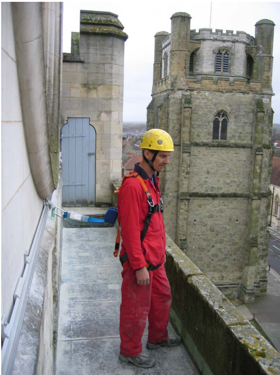
Unirail lifeline fitted to the North Nave Transept gable end, Chichester Cathedral.
